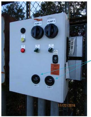
Photograph 1 – Pump run-time meters
